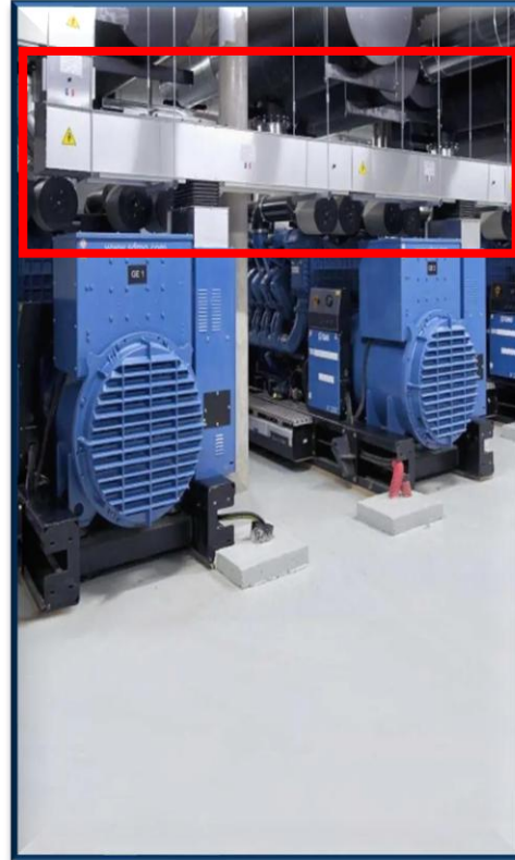
Diesel Generator to Synchronizing / Switchgear Panels
