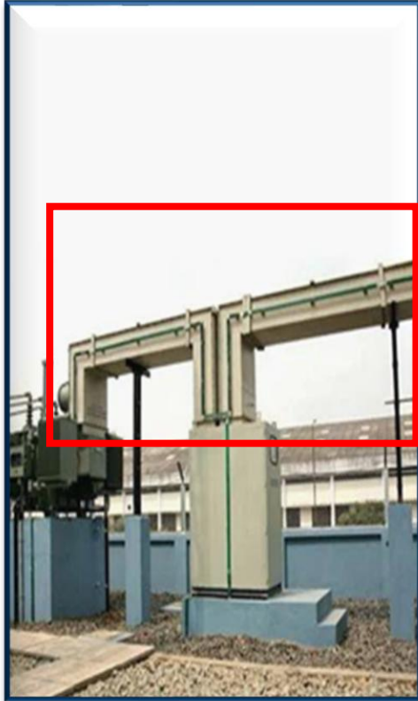
Interconnection between Switchgear Panels
