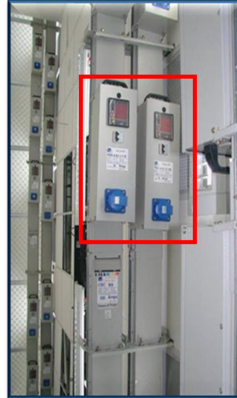
Rising Mains or Vertical Distribution in multi- storey buildings
