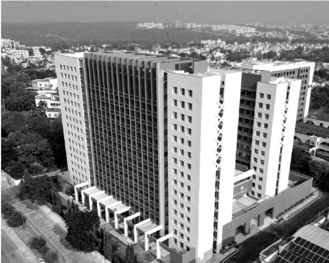
Hostel Building (1000 Students) for M/s Xavier Institute of Management , Bhubaneswar, Odisha.
