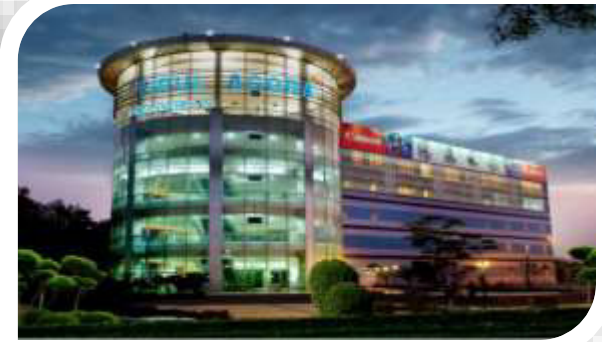
Vipul Agora MG Road, Gurugram Completed in 2006. Area 0.17 Mn. Sq. Ft.
