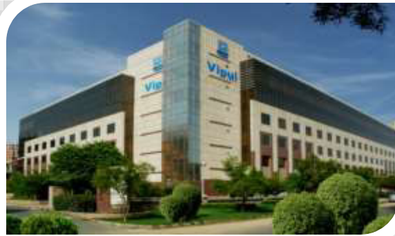
Vipul Plaza Sec 54, Gurugram Completed in 2005. Area 0.21 Mn. Sq. Ft.
