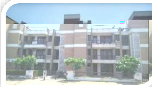
Vipul Floors Sec 48, Gurugram Completed in 2015. Area 0.09 Mn. Sq. Ft.
