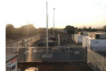
STATCOMs Upto 5 MVAR ratings
