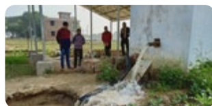
Installation of solar pump at Naini
