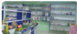
Renovation of High School Lab at Pallavaram
