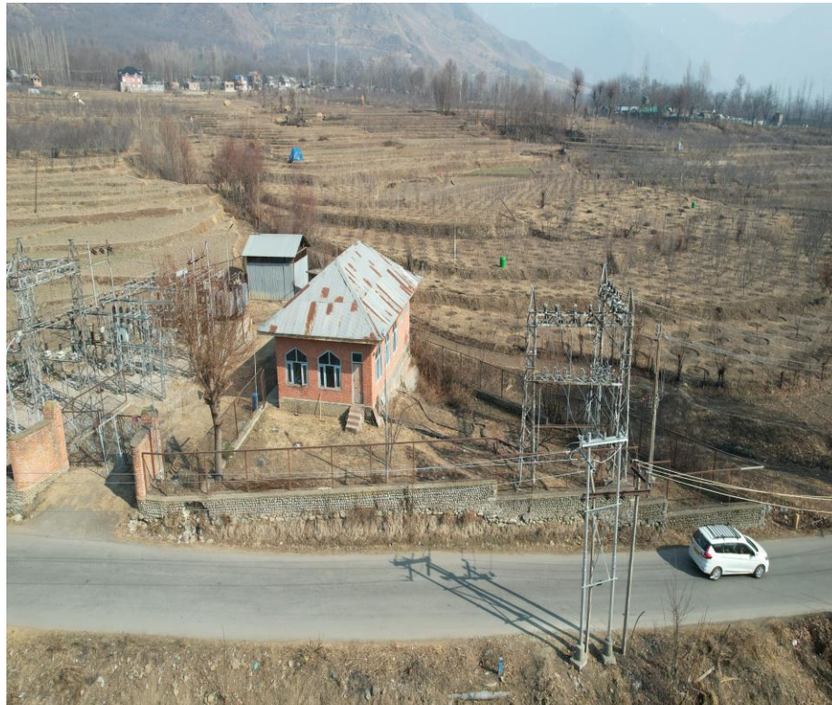
Loss Reduction project from PGCIL in Pulwama District, Jammu & Kashmir Status: On-going Line Length: 1,285 Ckm LT & 714 Ckm HT
