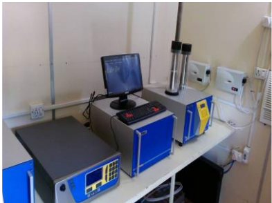
Online Continuous Air Quality Monitoring Station
