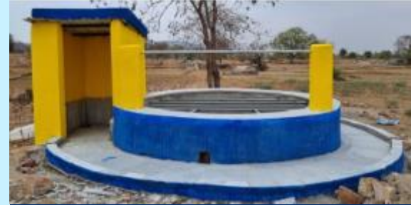
One of our renovated wells - Mahengro, Khaira
