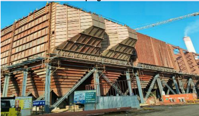
Unit #3 Electrostatic Precipitator Hopper erection work progress
