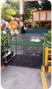
Wheelchair ramp @ APAR Umbergaon Cable Plant office entrance
