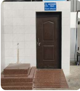
Washroom for specially-abled persons @ APAR Khatalwada Cable Plant
