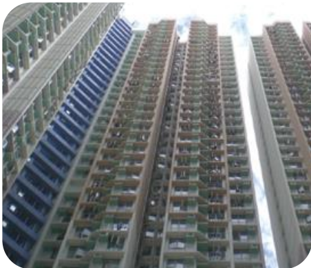
Breaking the Height Barrier
