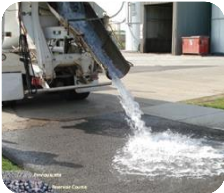
Instant Water Logging Solution
