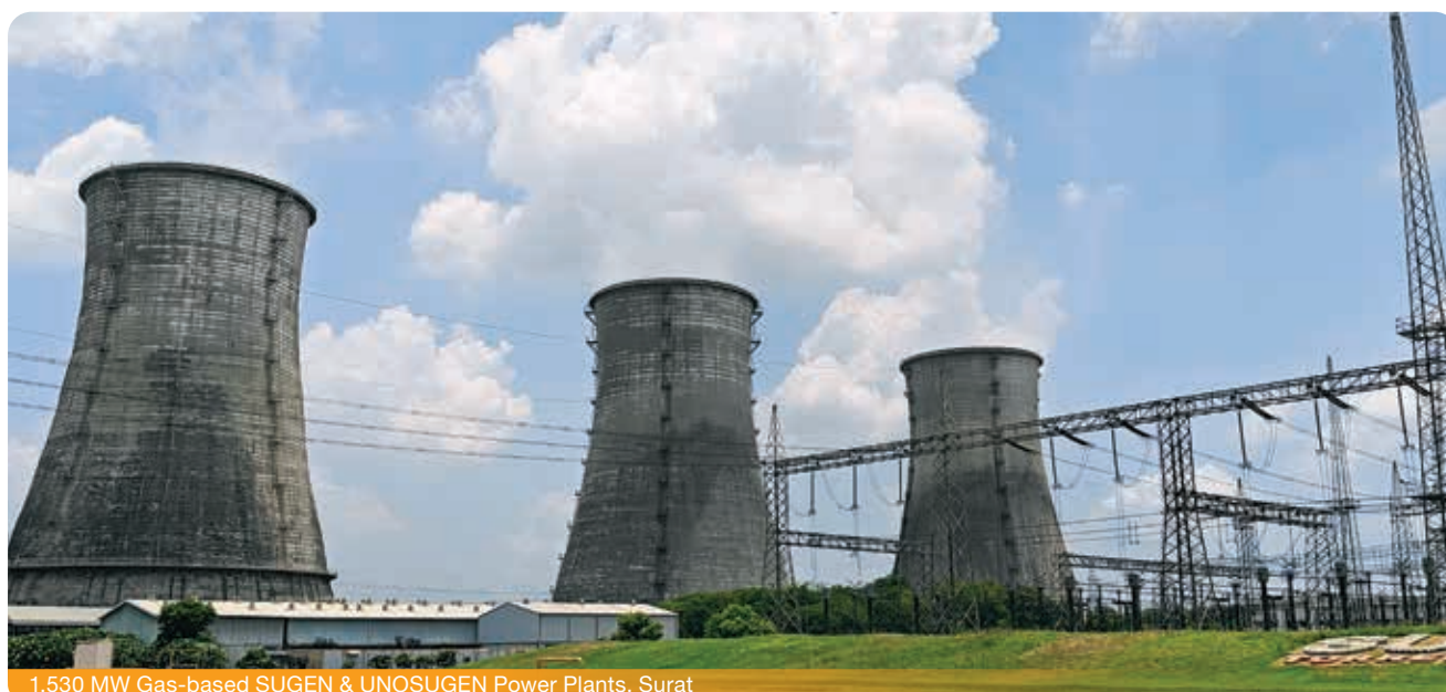
1,530 MW Gas-based SUGEN & UNOSUGEN Power Plants, Surat
