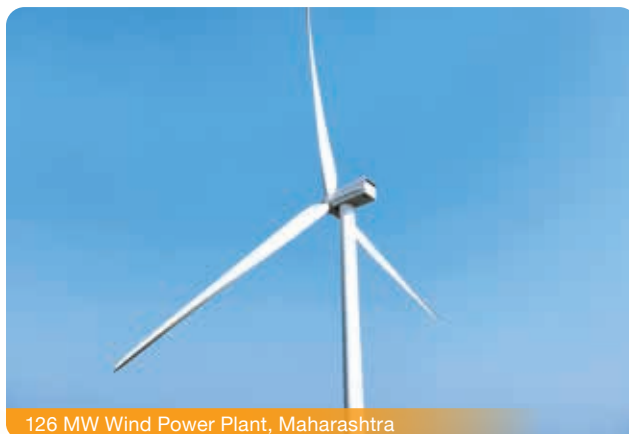
126 MW Wind Power Plant, Maharashtra
