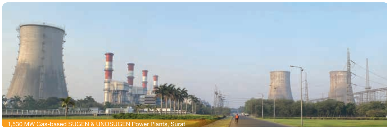
1,530 MW Gas-based SUGEN & UNOSUGEN Power Plants, Surat
