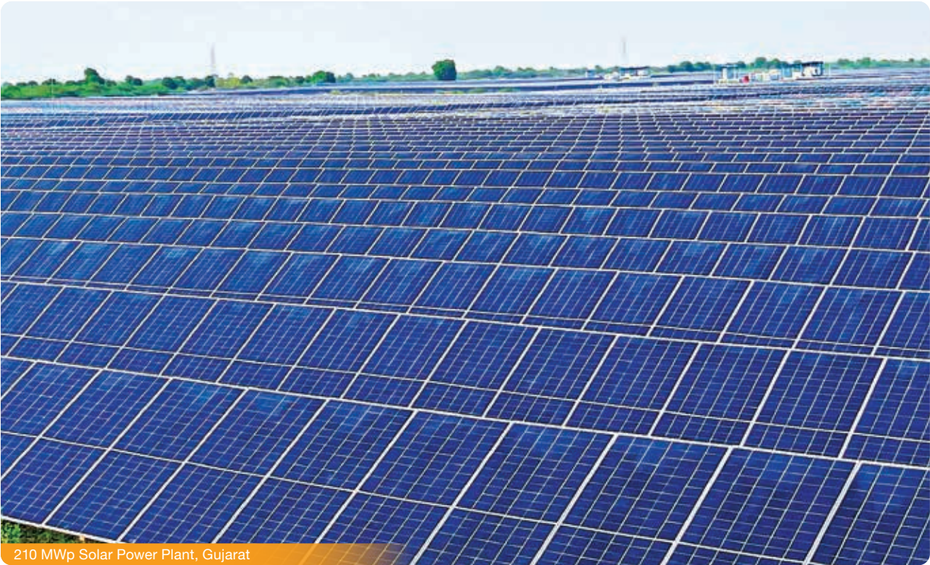
210 MWp Solar Power Plant, Gujarat
