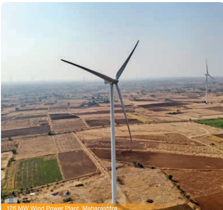
126 MW Wind Power Plant, Maharashtra
