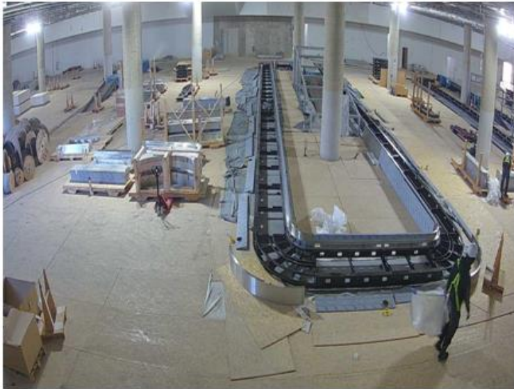
Terminal Building Baggage Handling works at Arrival Hall
