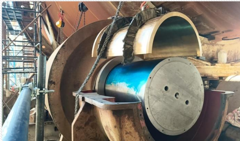
Kiln support roller bearing scrapping work in progress
