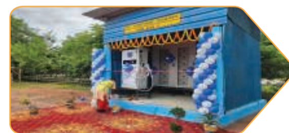
In House EV Charging Station
