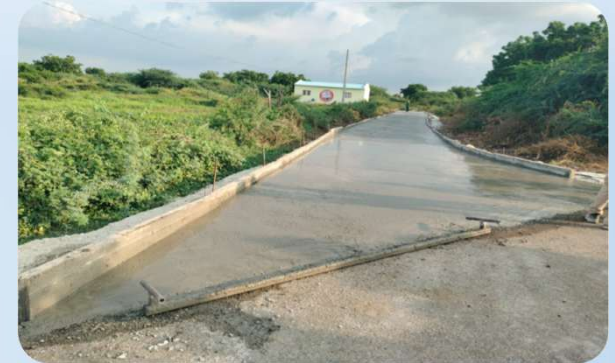
Laying of CC Road At Ramapuram Village, Dacheipalli, Andhra Pradesh
