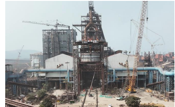
BF-3 upgradation project at Vijayanagar
