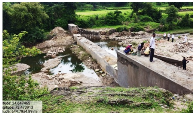
Water harvesting structure (anicut) in Udaipur, a water scarce region in south Rajasthan
