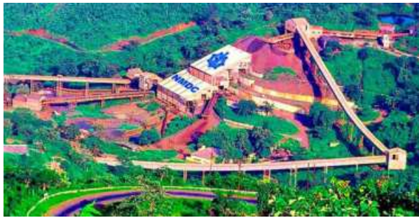
CAPEX PLAN. Nearly ₹12,000 crore worth of expansion projects are underway and expected to be completed over the next three years
