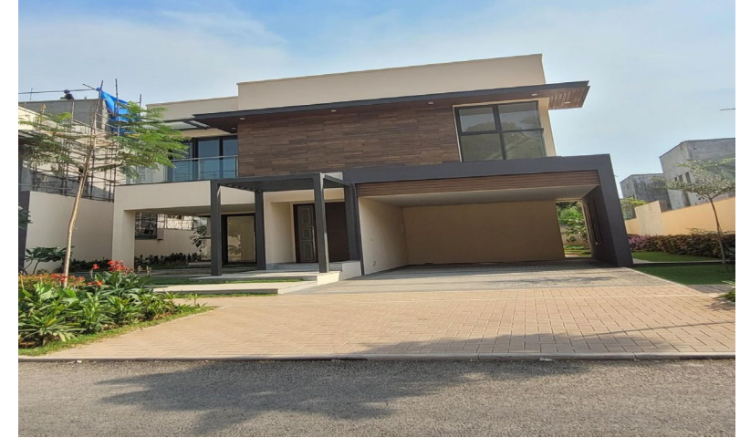
SOBHA Silver Estate Thrissur
