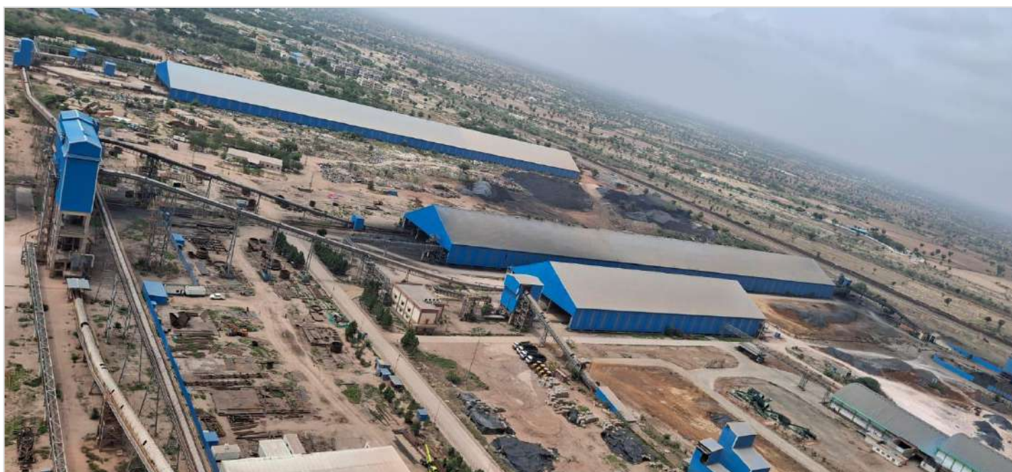
Exhibit 5: Storage facilities for limestone, coal and gypsum
