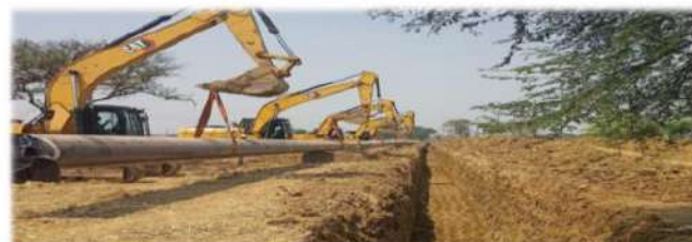
Setting up slurry pipeline
